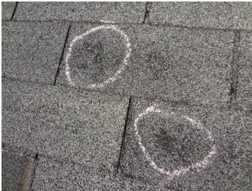
Hail hits are black in color due to loss of granules, which may expose the roof felt.
